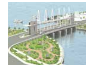
Facilities to prevent salt water intrusion (Image for illustrative purpose only)
