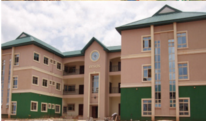
Anambra State University teaching hospital in Awka, which is nearing completion
