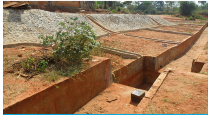
Completed intervention at Ebenebe gully erosion site
