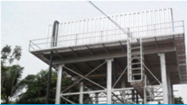
An ongoing Udoka water project in Awka
