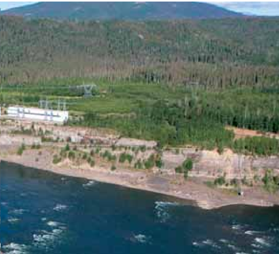
Above: the Peace Canyon Dam and powerhouse, British Columbia. BC Hydro provides energy solutions in an environmentally friendly way
